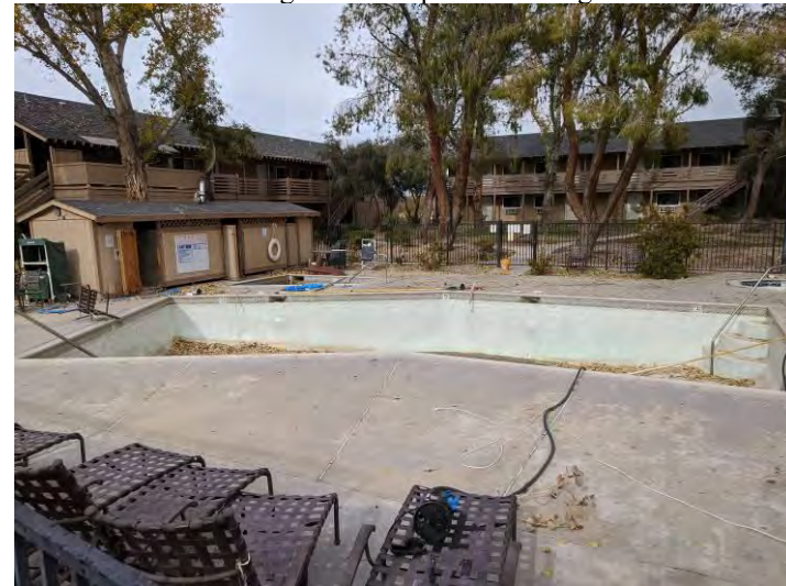
One of two swimming pools next to clubhouse
