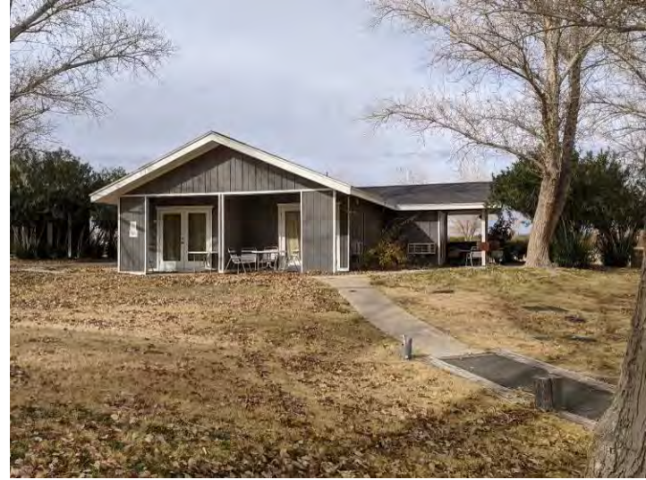
Four-unit Bungalow building (one of two)
